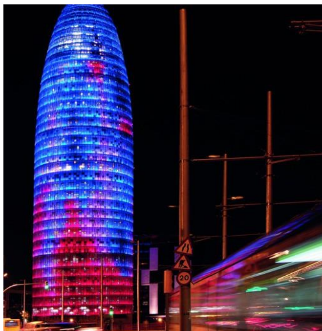
GLORIES TOWER VIEW POINT
